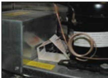
Figure 3. Monitors for pest activity inside of kitchen equipment.
